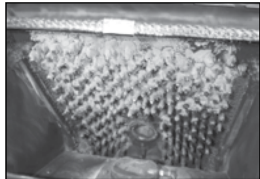
Figure 35.2 - Example of a dirty heat exchanger
